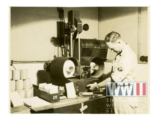
Letters are printed onto large rolls of paper and inspected for quality. If an image did not develop well, it was marked out and re-processed.
