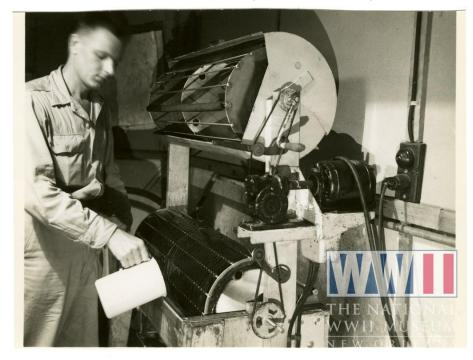
The developed film is enlarged from about the size of a thumbnail to  $4\,\%\,x\,5$  in.
