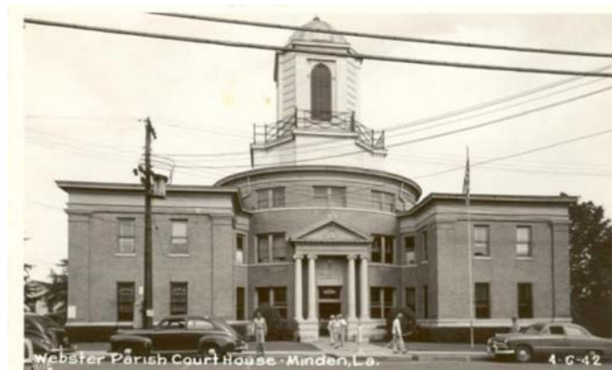
Webster Parish Court House, Minden, Louisiana. Courtesy of courthousehistory.com
